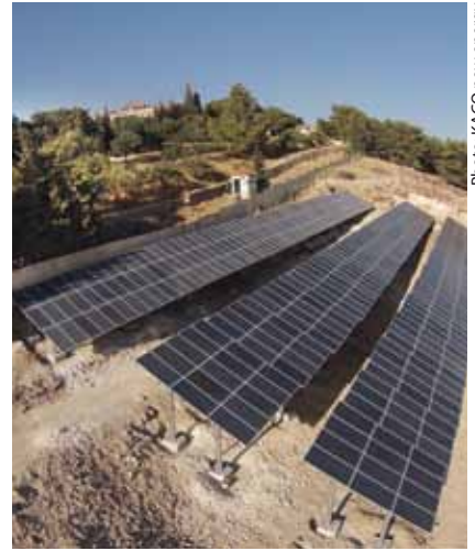
Photo: KACO new energy
